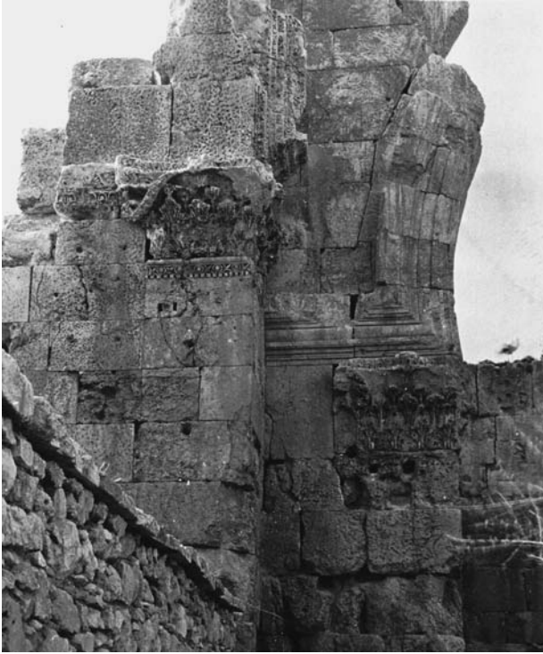
Fig. 2.6.3 Basilica, part of apse archivolt and south-eastern corner of the nave Source: Gertrude Bell Archive, Newcastle University, S 176.
